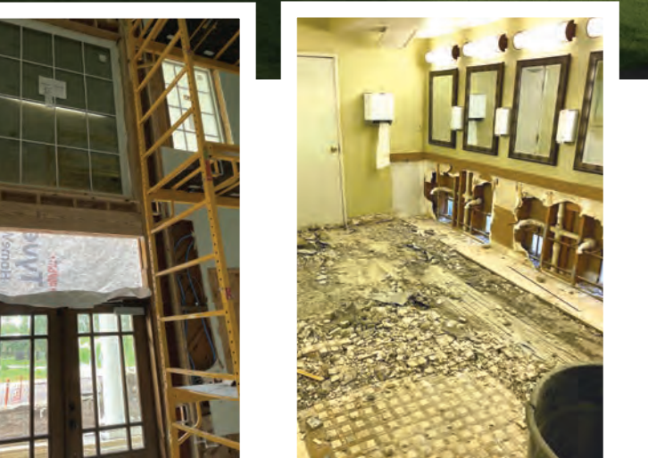
Above: Interior house renovations in the summer 2023.
